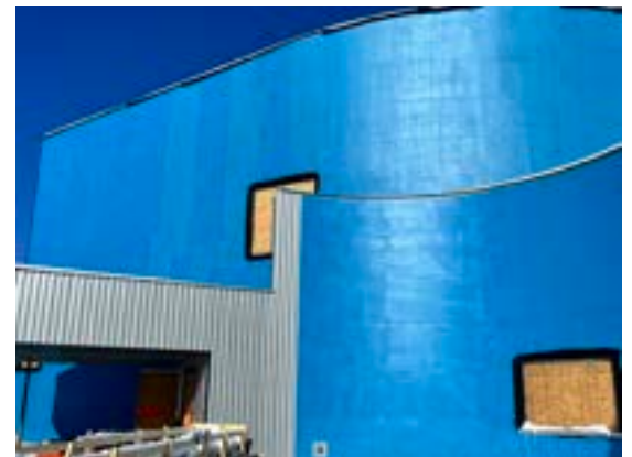
The beginning of the metal cladding that will cover the building.
